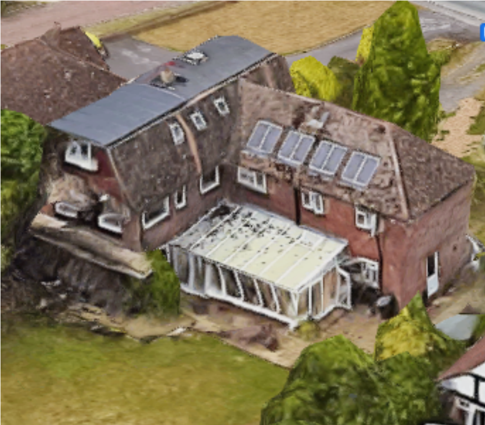
Figure 4: Exmample of a gambrel roof form approximately 80m to the west (no.6).
